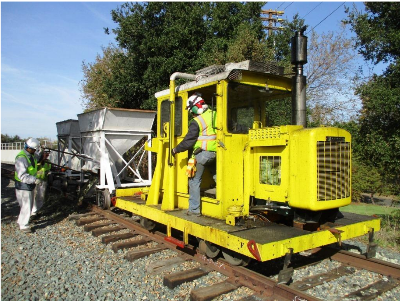
Joe skillfully pilots the Kalamazoo as Mike H. and Jose discharge rock from the side-dump cars
