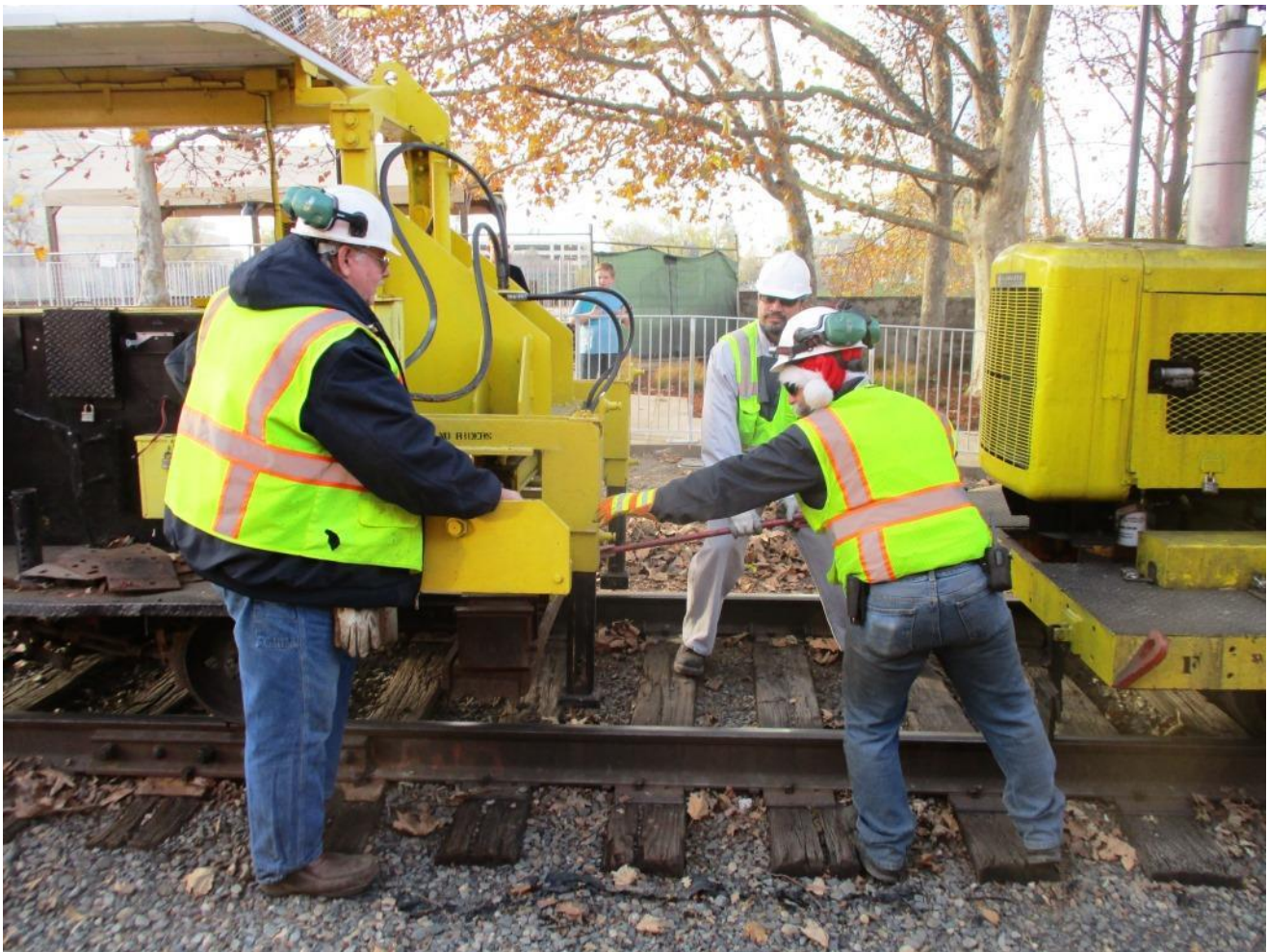
Chris, Jose, and Joe now hook the 125 to the Kalamazoo to be pulled over to the Shops
