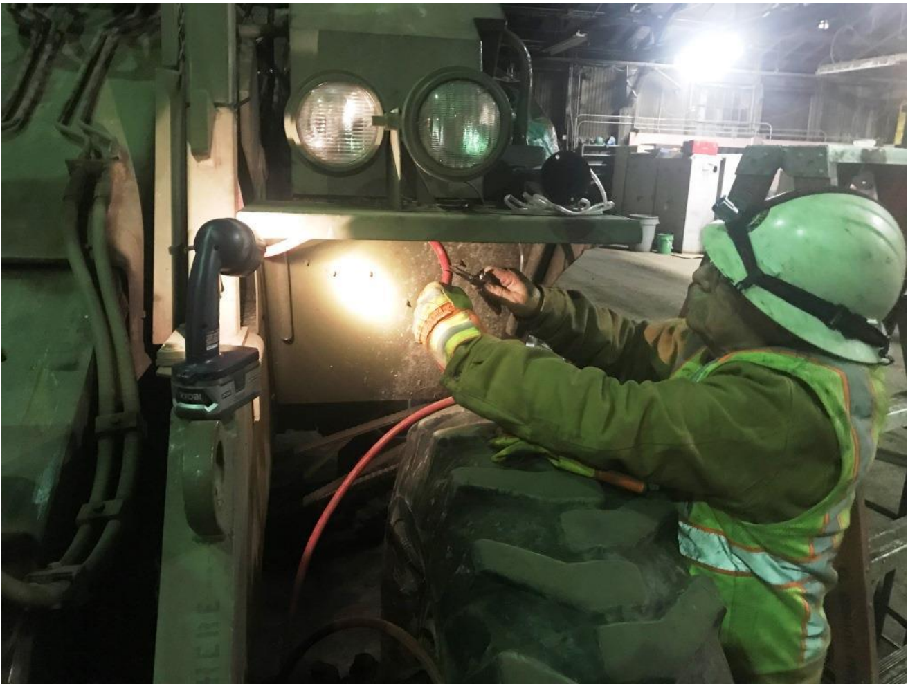
Mike H. finishes plumbing the air-lines for the new horn on GM2
