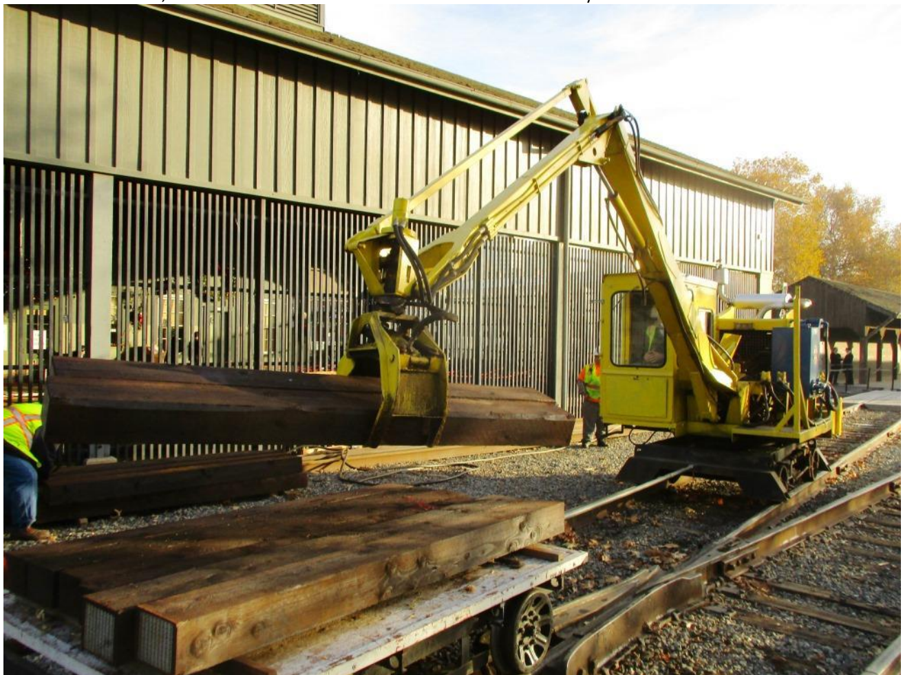
Ties, ties, everywhere! Alan loads them onto a flatcar
