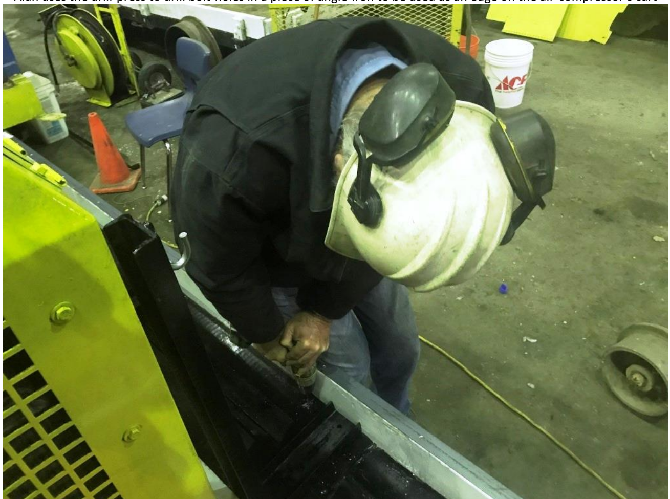
Alan drills bolt-holes through the deck of the compressor's cart where the new mounting brackets will be attached
