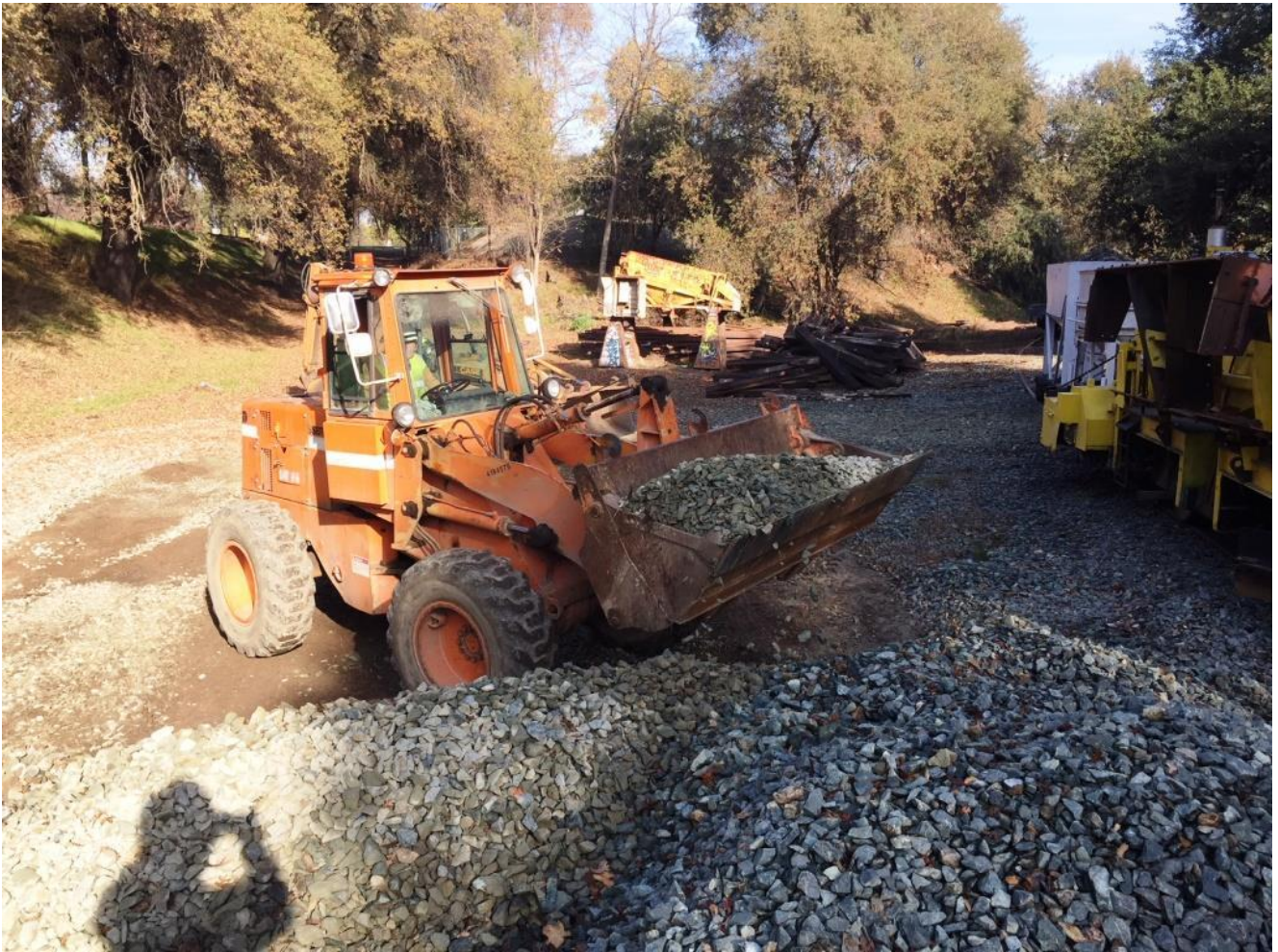
At Setzer, Mike H. in the loader scoops up a bucket-full of rock
