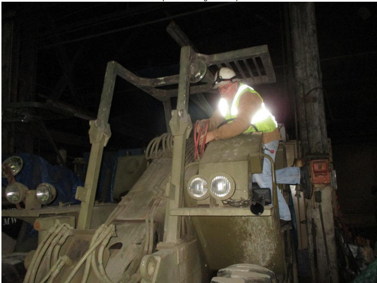
Mike H. plumbs an air-line for the new horn on GM2
