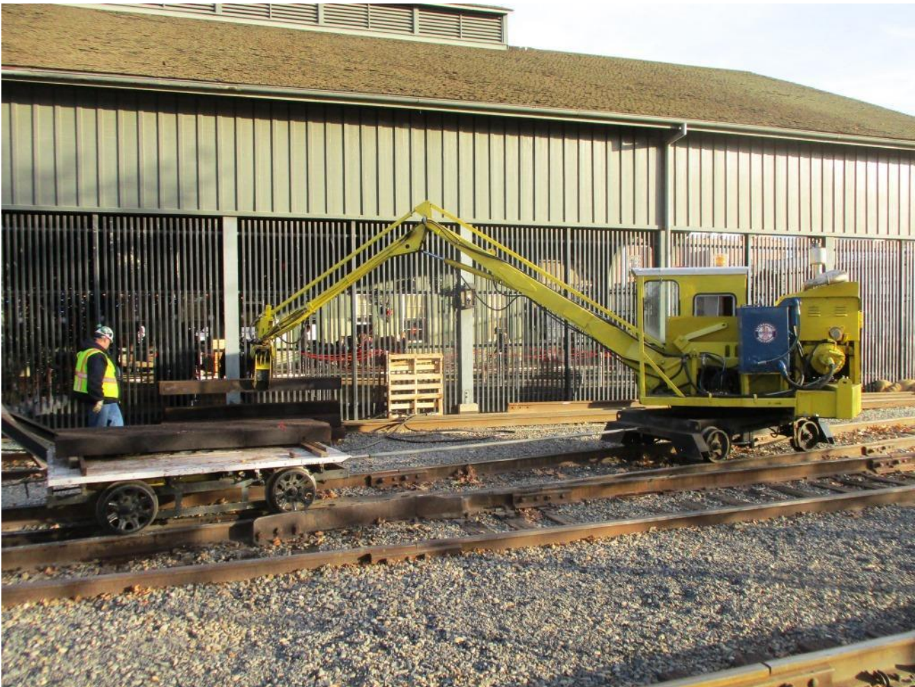
Meanwhile, Alan in the tie-crane moves the bundle of ties stacked by the south end of the container
