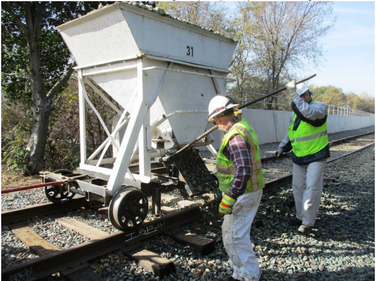
Mike H. and Jose discharge rock from the side-dump car
