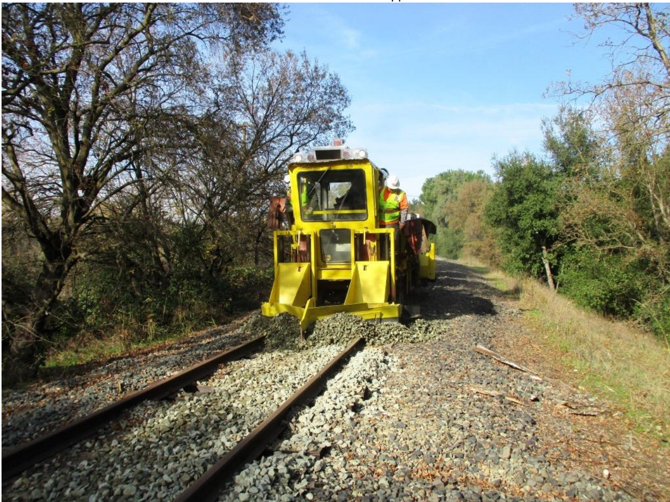
After the rock is disgorged, Chris in the ballast regulator plows the track and spreads the rock
