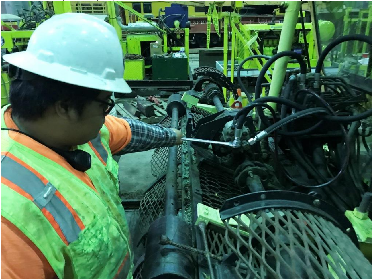
Anthony installs new hydraulic lines on the scarifier
