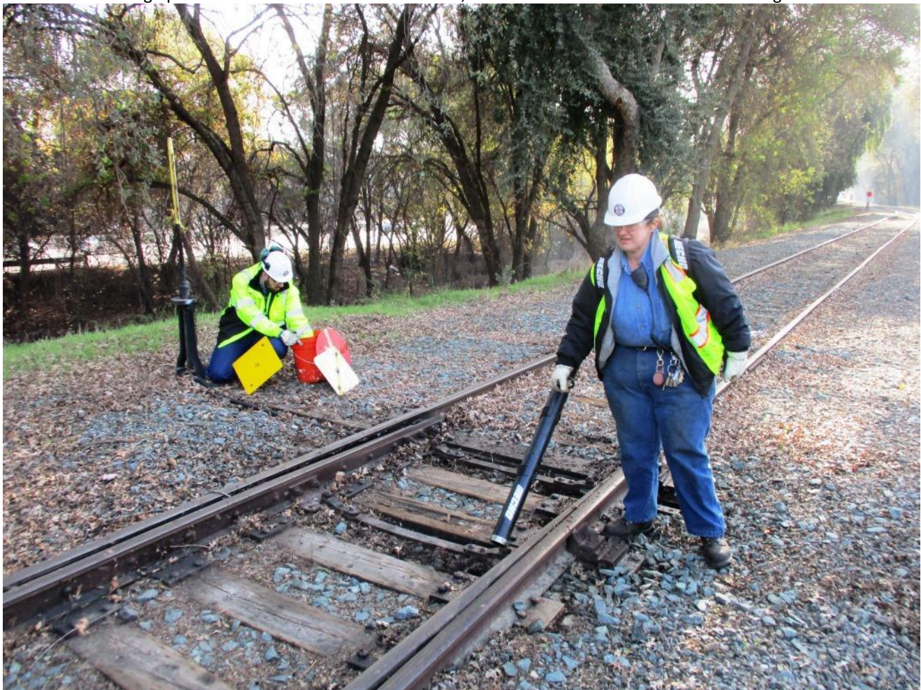
As Weston replaces the target at Switch 15, Heather takes the opportunity to remove organic debris from the track
